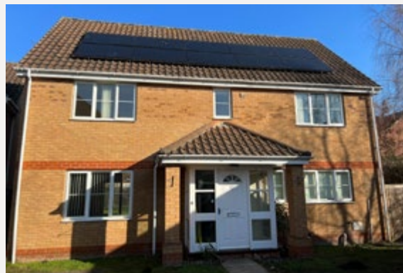
A home in the Mildenhall development, fitted with solar panels
